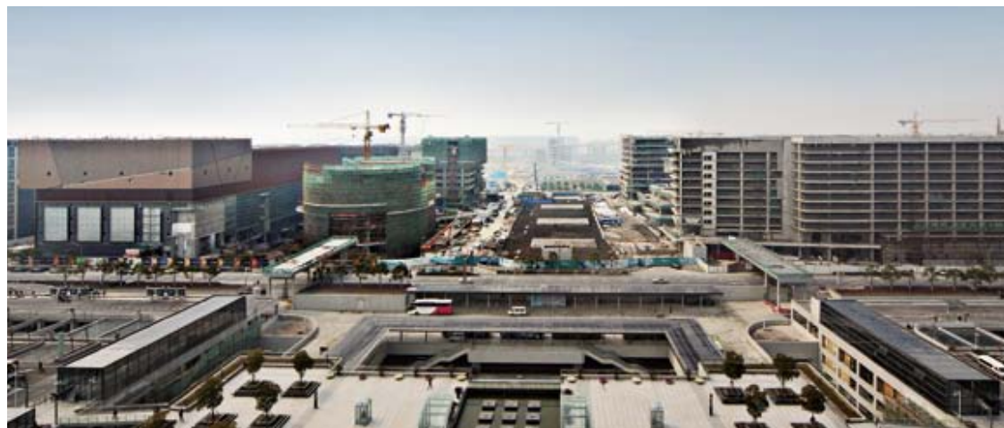
◀ Construction site of THE HUB
