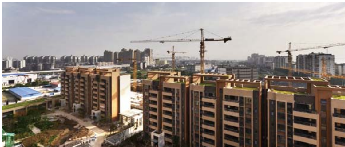
◀ Construction site of Wuhan Tiandi
