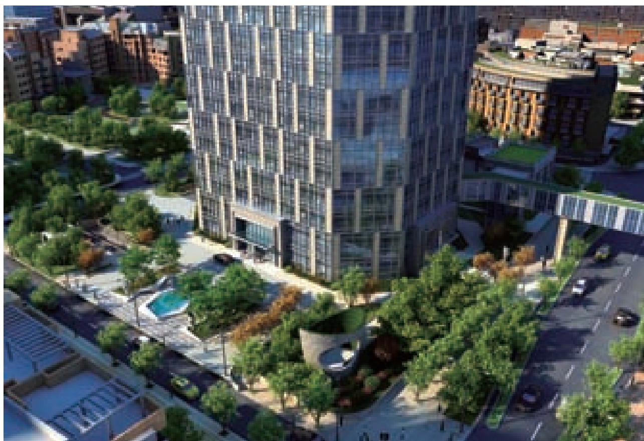
Lot A5, office building in Corporate Zone at Wuhan Tiandi
