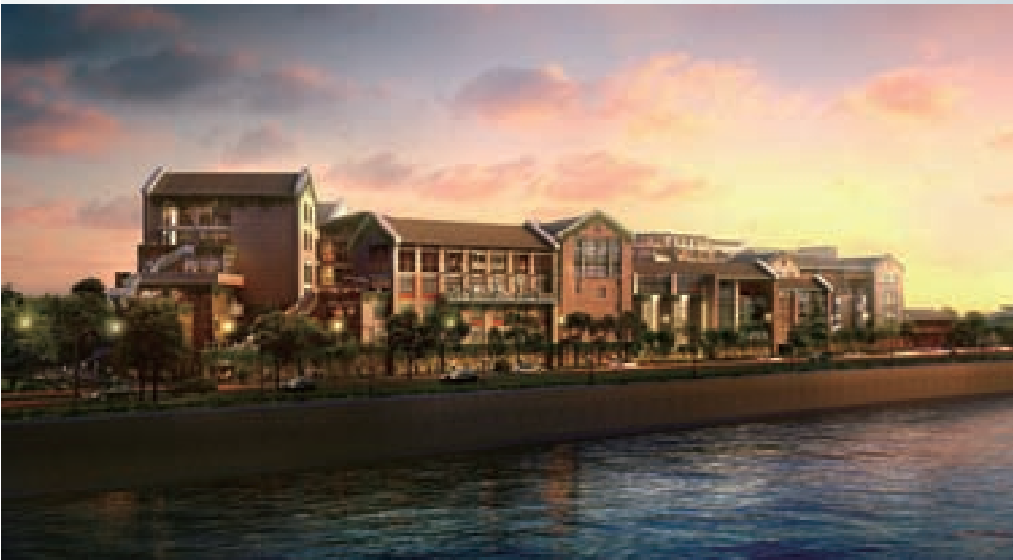
Architectural tradition "Cliff Building" featured at Chongqing Tiandi
