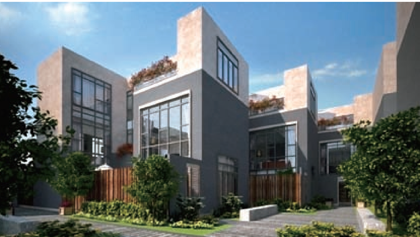
The residential area at Foshan Lingnan Tiandi
