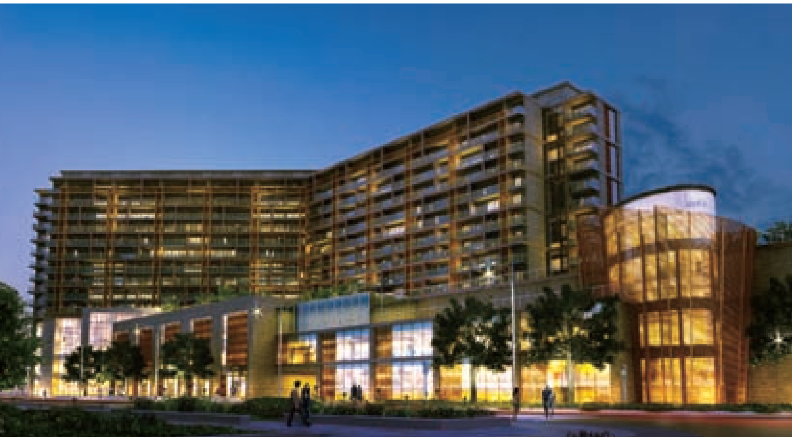
Lot D, the service apartment and shopping centre at Foshan Lingnan Tiandi
