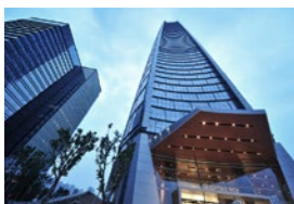
Chongqing Xintiandi, A Hall and B Hall of Jialing Mall and 2 Corporate Avenue Retail, Chongqing
