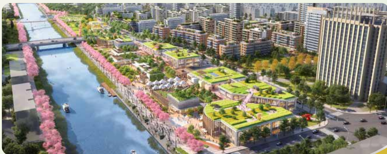
Fengxian Beigang City Village urban regeneration project
